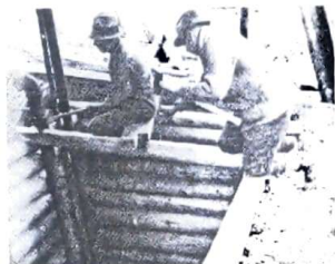
Rebuilding Shaft Collar at No. 1 Shaft
