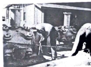
Unloading 1050 cu. ft. Electrically Driven Compressor
