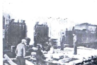
Placing Main Transformers at Power Line
